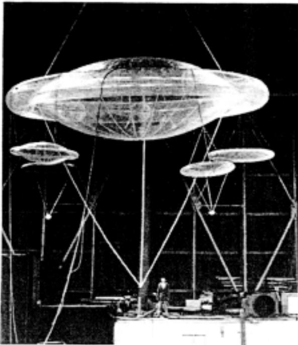
Figure 3. Lenticular Inflatable Parabolic Reflector
